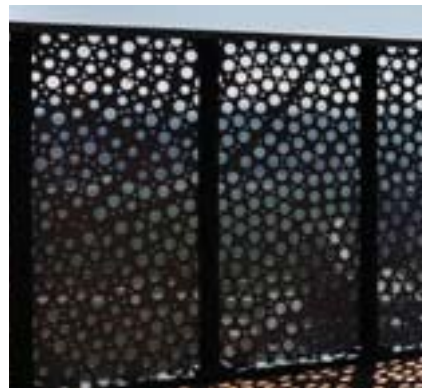
PERFORATED METAL - GUARDRAIL & INFILL PANEL
